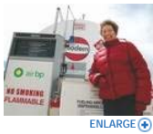
Kay Bennett, co-manager of the Silver Springs Airport, stands next to a new fueling station at the airport that will be dedicated next week. Brian Duggan/Nevada Appeal
